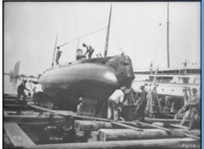
USS Holland (SS-1) Construction
