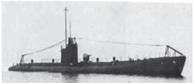
The RO-33 showing bow anti-submarine net cutter.
