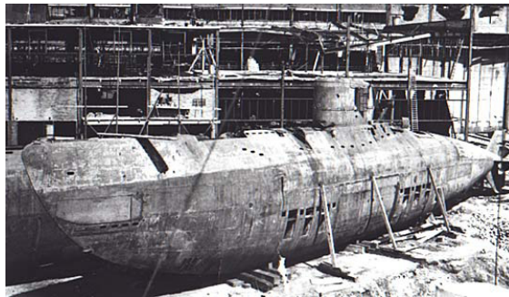
The Type Wa-201 Walter boat, U-793, here partially dismantled at the end of the war.
